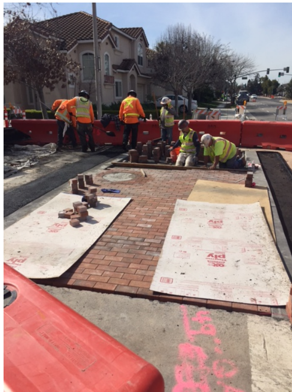
Center section of paver crosswalk at Frances/Iowa being installed.
