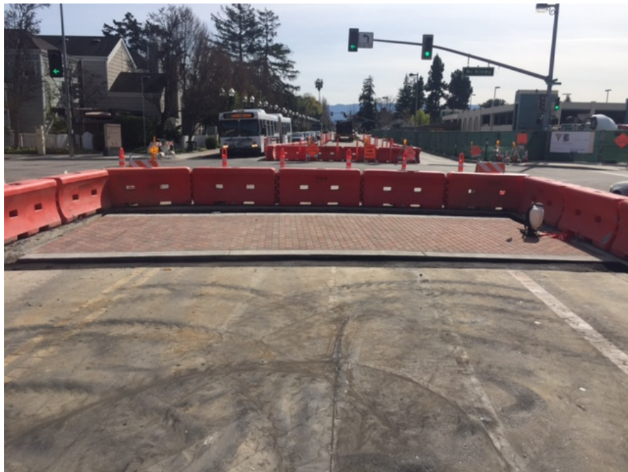
Center section of paver crosswalk at Sunnyvale/McKinley complete.
