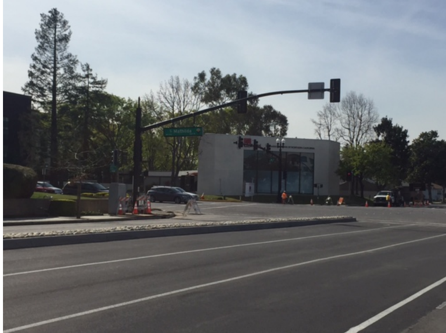
New traffic signal poles at Mathilda/Iowa erected.
